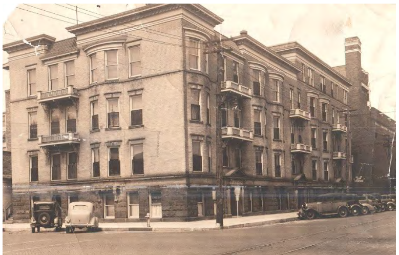
Above: Façade pictures of the Sala building in 2005 and circa 1920. Below: Interior photos of Sala Flats apartments. Refinished balconies on the west side of the building.
