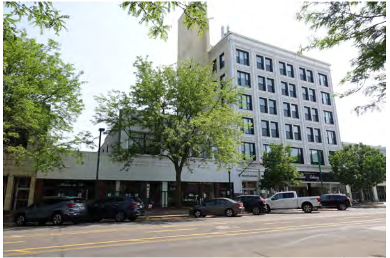
Above: Wilson Lofts is the tallest building in Clinton, IA.
